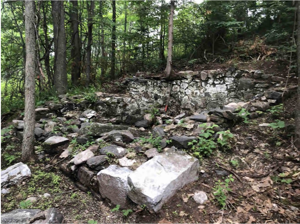
Photograph 25: Foundation 2. View north
