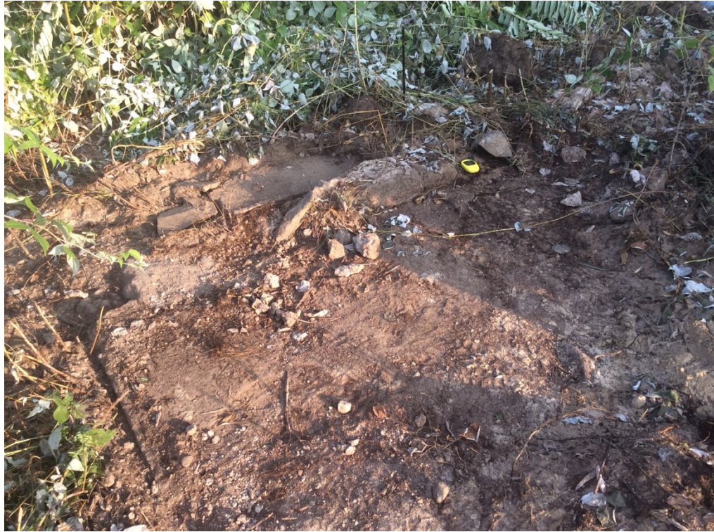
Photograph 17: Foundation 3 - poured concrete.
