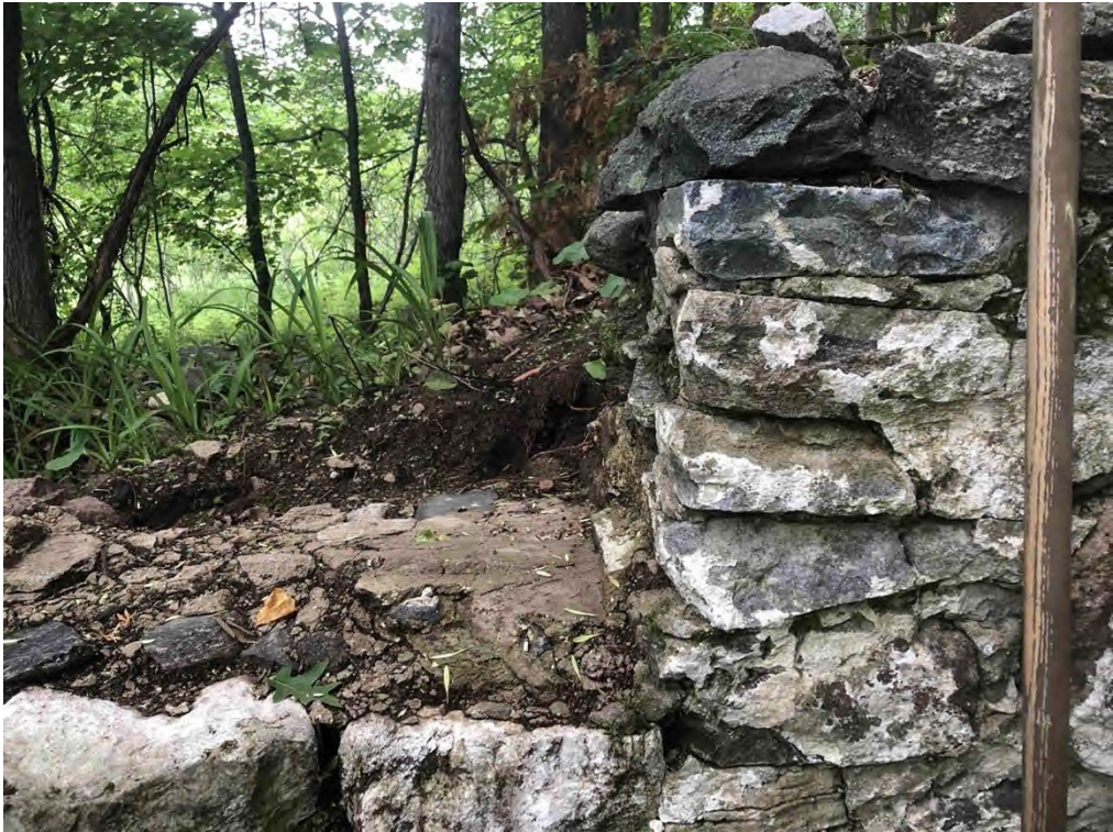
Photograph 26: Foundation 2. Window reveal.
